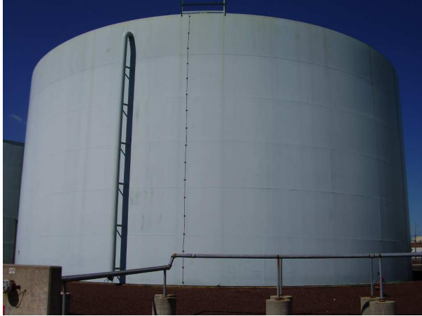
3.0MG Steel Standpipe in CT 78 ft dia. by 80 ft tall
