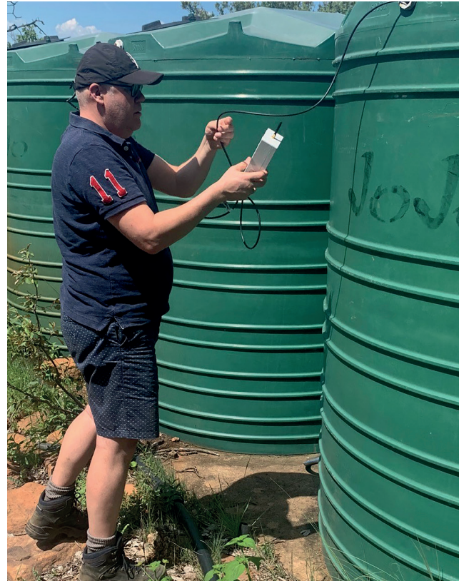
Installing the level sensor and LoRa modem
