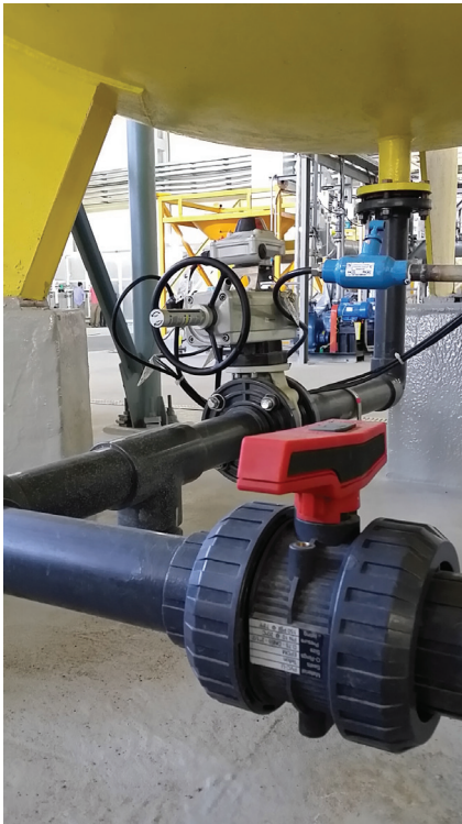
Mining and metalurgical plant RUSSIA
