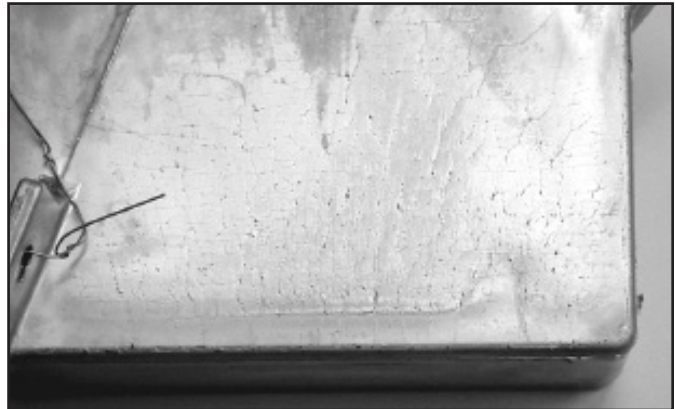
Figure 2-14 Washout as seen on a casting.
