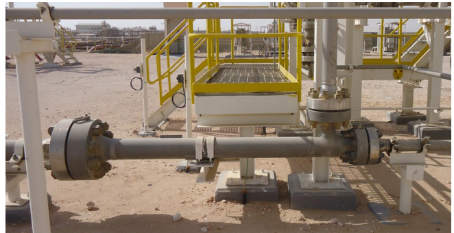
LJC to recover waste flare gas, installed in Oman
